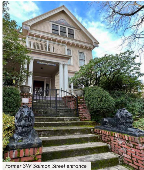
SW King Street entrance
