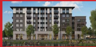
Henley Place Apartments 178 Units | Opening 4/2024
