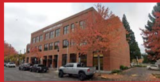
New Milwaukie City Hall 10501 SE Main Street
