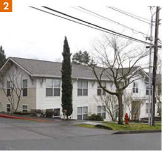
6171 SW CAPITOL HWY Portland, OR 97239
